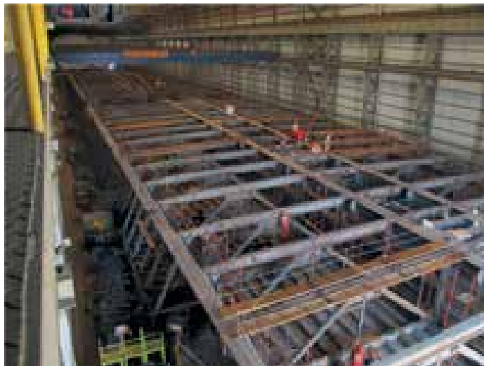
12 Geometriekontrollen im Werk in Shanghai © Forth Crossing Bridge Constructors
