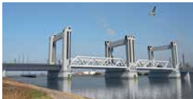
■ Botlek-Hubbrücke in Rotterdam © Konsortium A-Lanes
